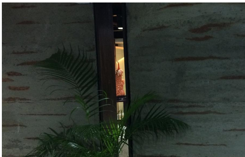
Fig. 3. The rammed earth wall of the high-rise building
