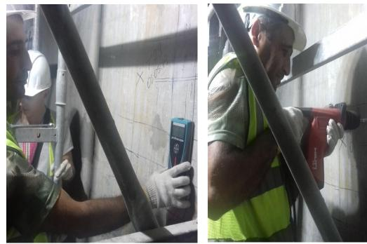
Fig. 5(a). Usage of Rebar Locator.
