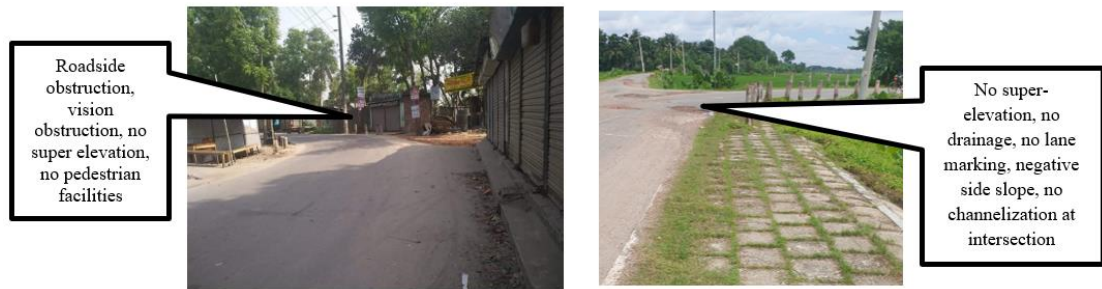
Fig. 3. & 4. Sharp curve, no super-elevation, drainage, negative shoulder slope, channelization, pedestrian facilities of common rural roads.
