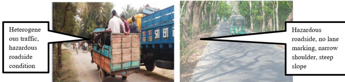
Fig. 1. & 2. Roadside hazardous, traffic characteristics, narrow shoulders of RRs
